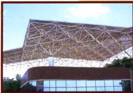
IOCL Refinery, Baroda
