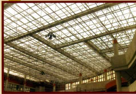
IOCL Refinery, Baroda
