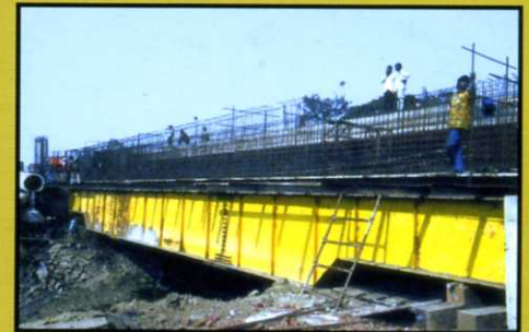
Launching Girder, RBM PATI, Kolkata
