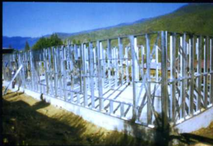
Cold form Structure for School Building
